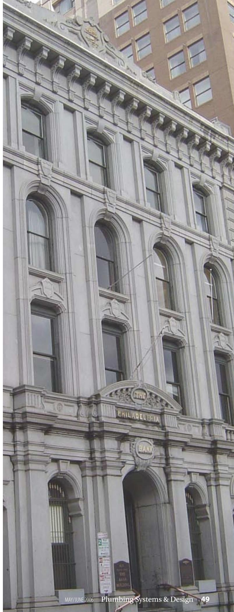
**Figure 3** In the existing historic area, the cement open structure with plaster architectural details limited the amount of pipes passing through open areas.
